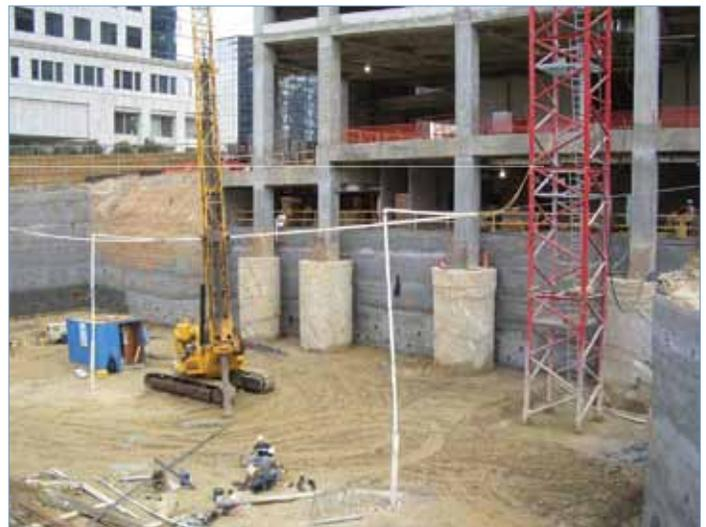
Combined Tower Column/Drilled Pier.
